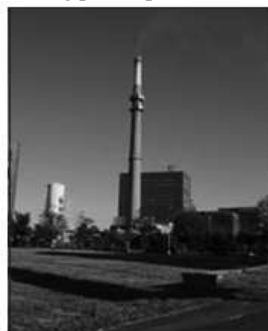
Locals would like to shut down the Fisk Generating Station at 1111 W. Cermak Rd.
