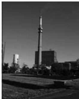
Locals would like to shut down the Fisk Generating Station at 1111 W. Cermak Rd.
