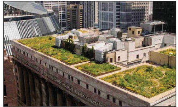
The Chicago Green Roofs Grants program provides grants for those building environmentally beneficial roof top gardens.
